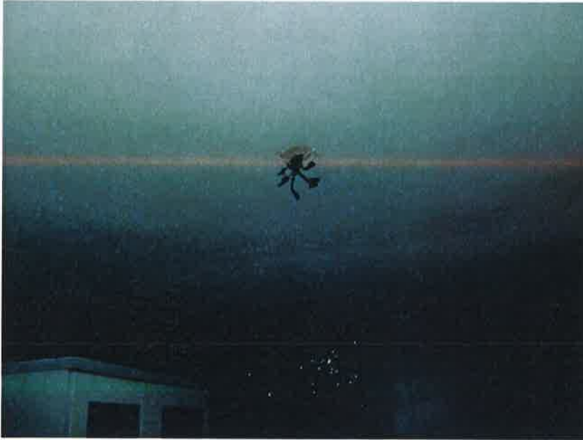
Missing light fitting in kitchen – December 2016
