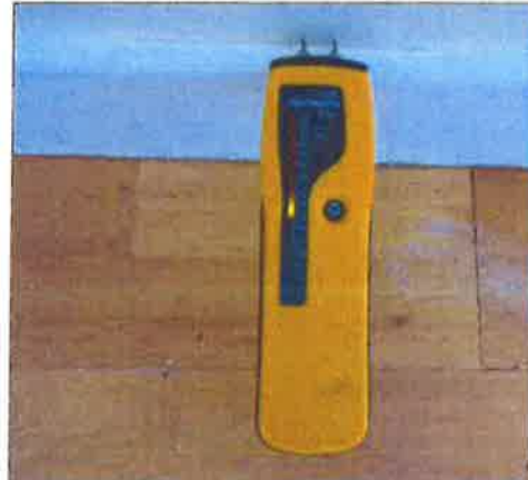
Picture taken 12/1/18 bedroom 1
