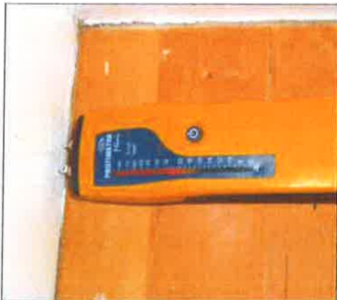
Picture taken 31/3/17 bedroom 1
