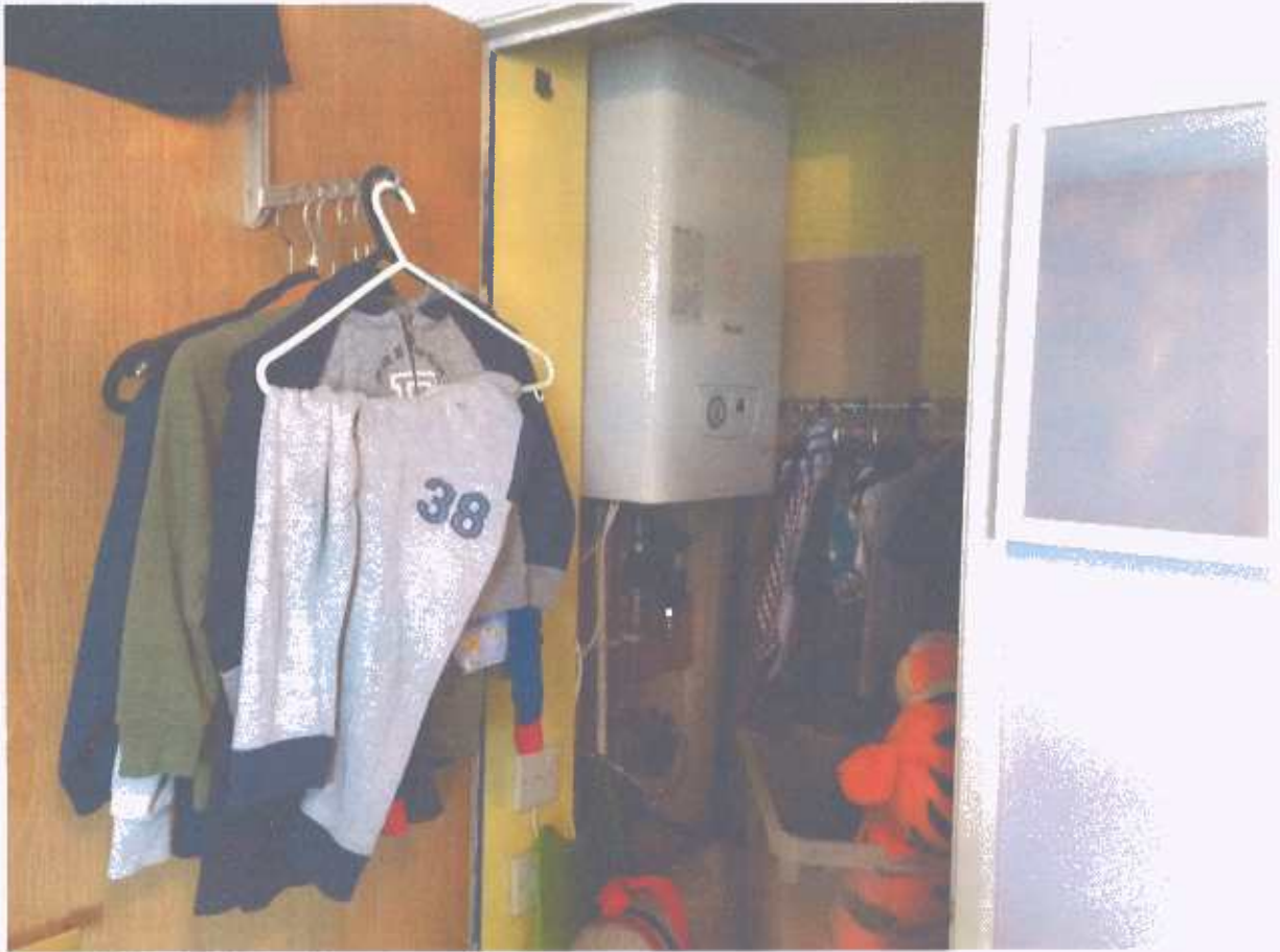
View of the first floor bedroom boiler – no ventilation via the door and no carbon monoxide detector in the bedroom
