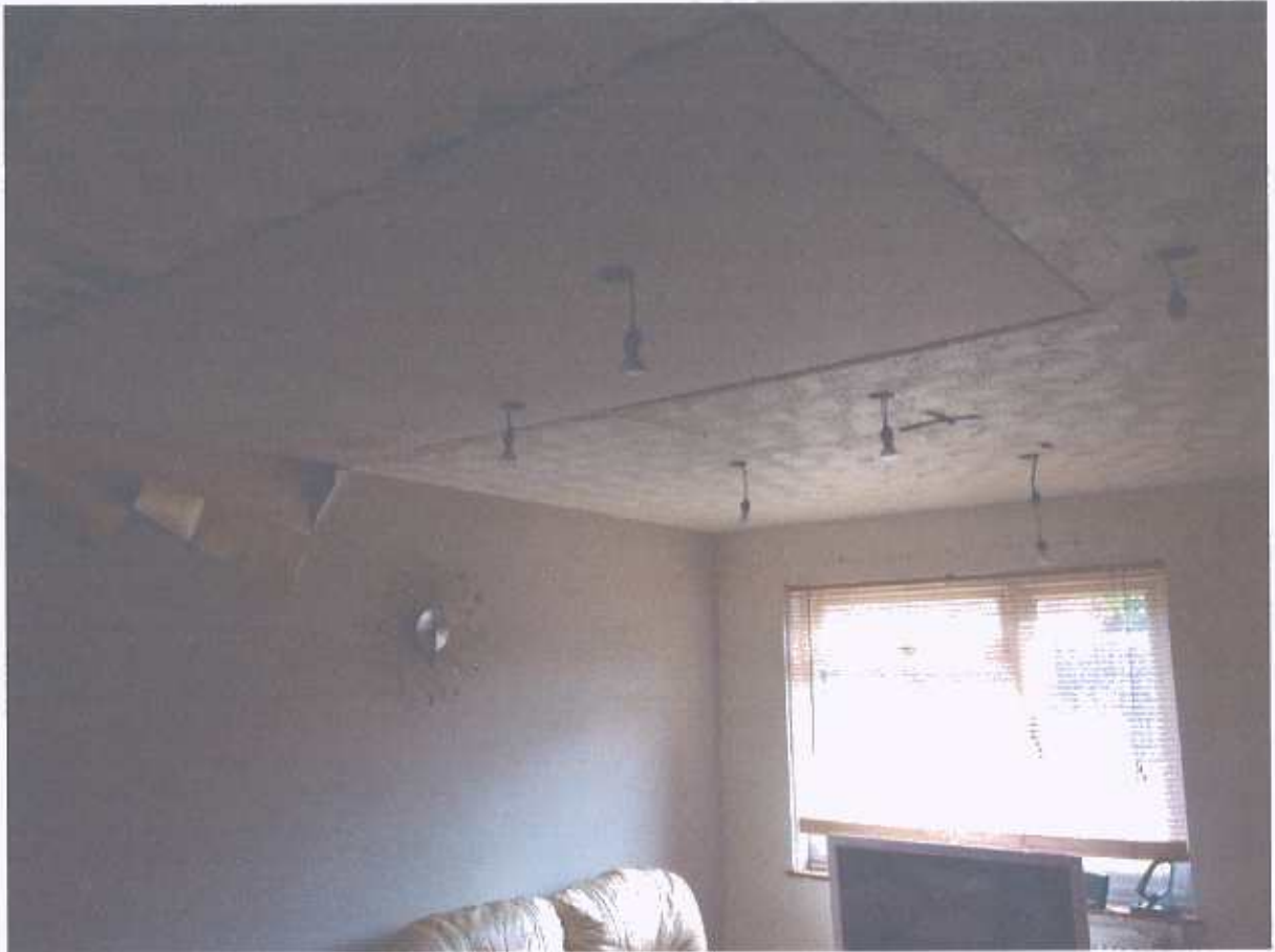
View of the unfinished ceiling repair, the hanging spot lights and the water damaged wallpaper
