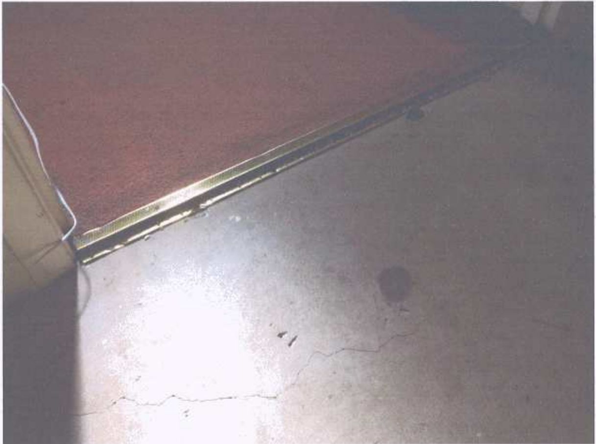
View of the exposed threshold carpet gripper strip at the living room entrance
