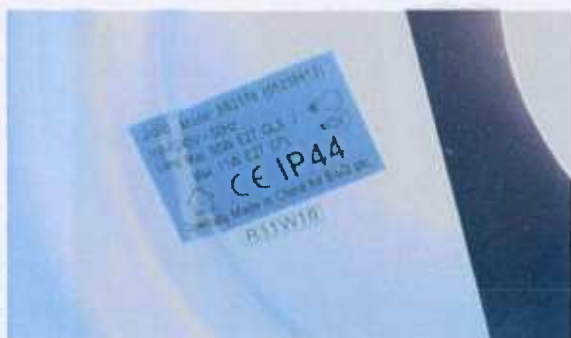
(Ph10) B/R – C/L not suitable for room
