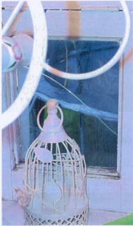
(Ph11) H/C – Cracked glazing
