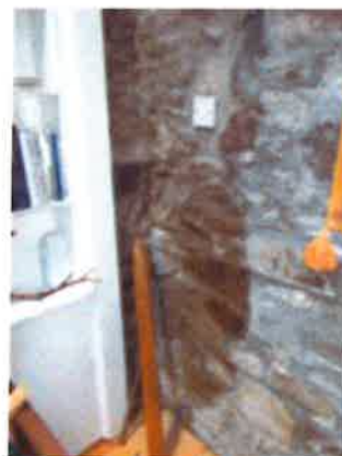
Communal Hall - large damp stain to rear stone wall.
