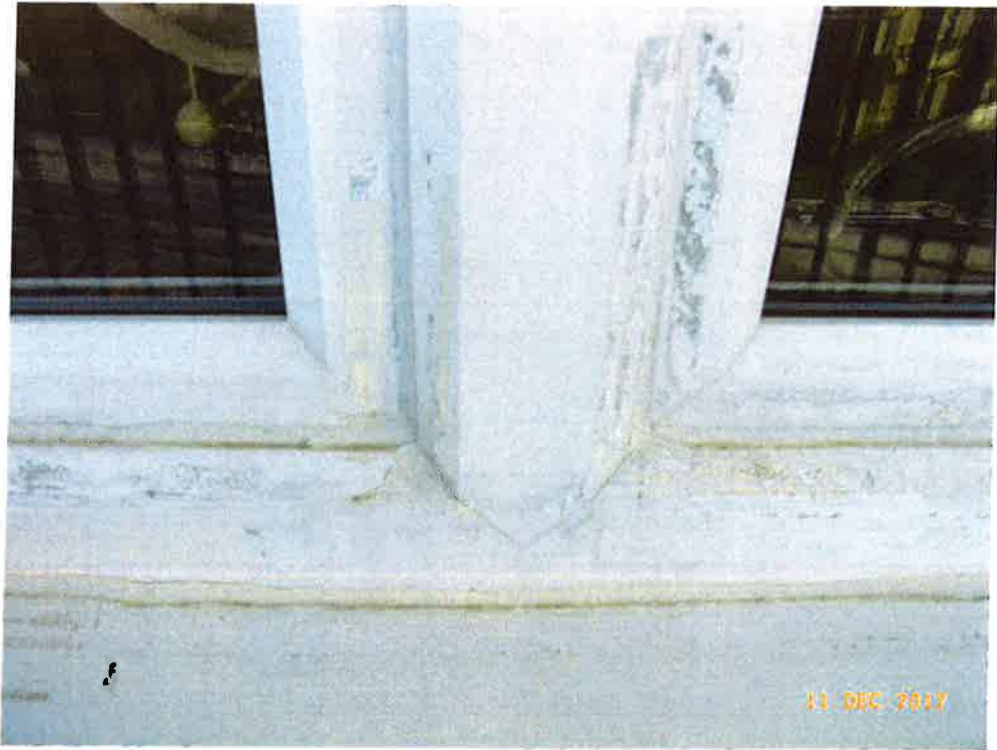
Lounge window exterior (2)
