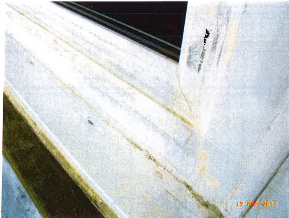
Lounge window exterior
