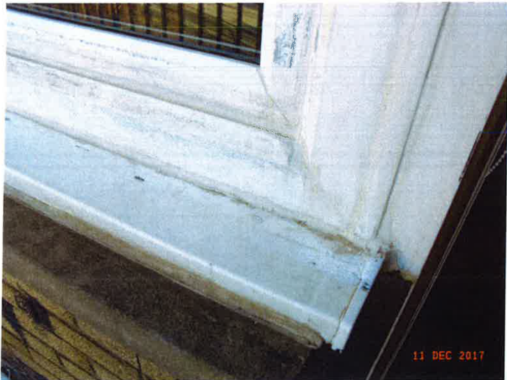
Lounge window exterior
