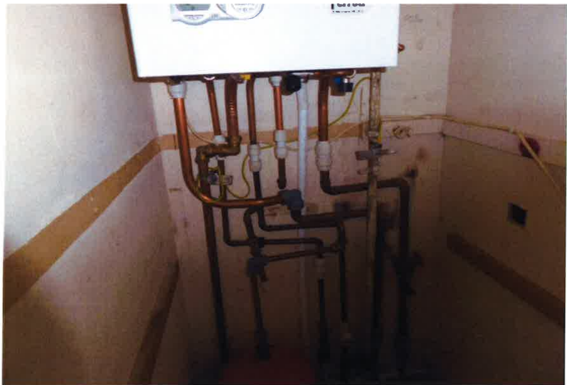
Central heating boiler pipework
