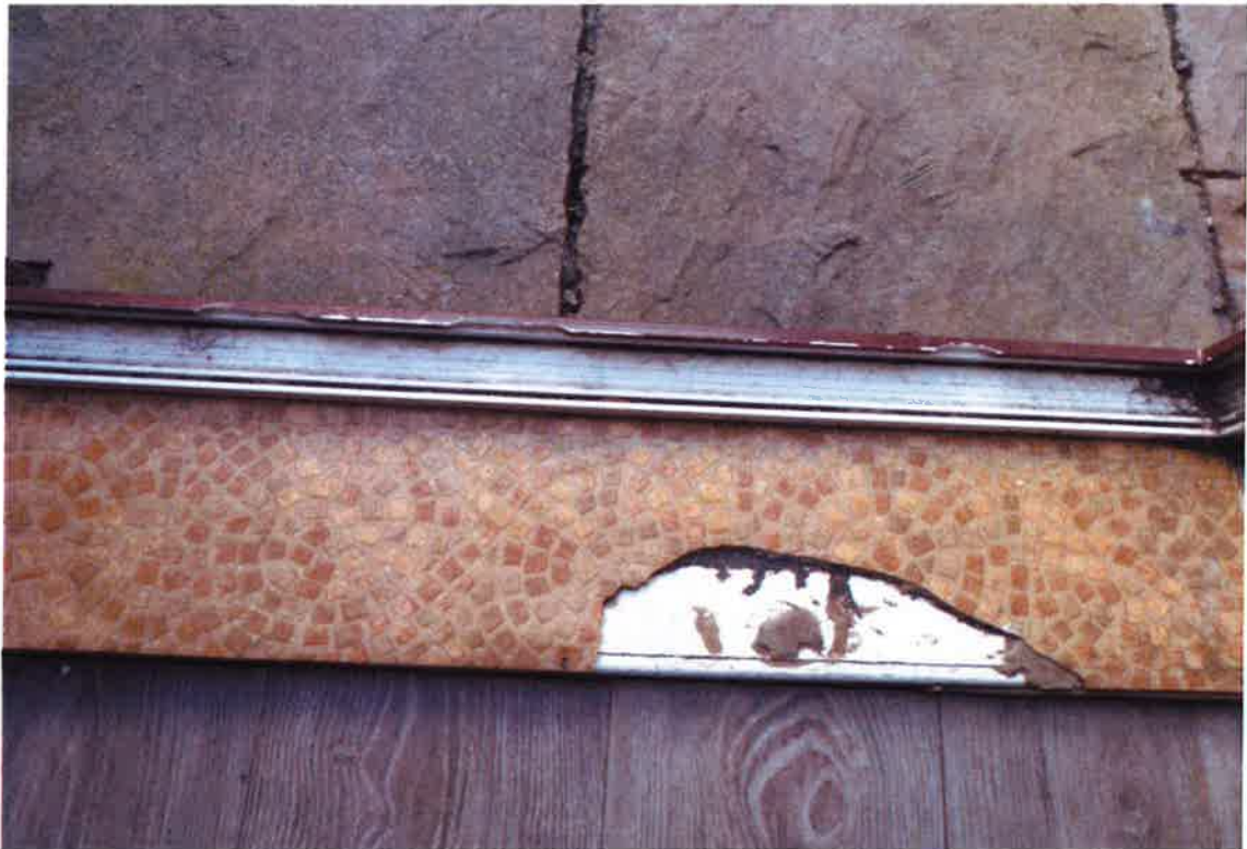
Rear door showing damaged sill
