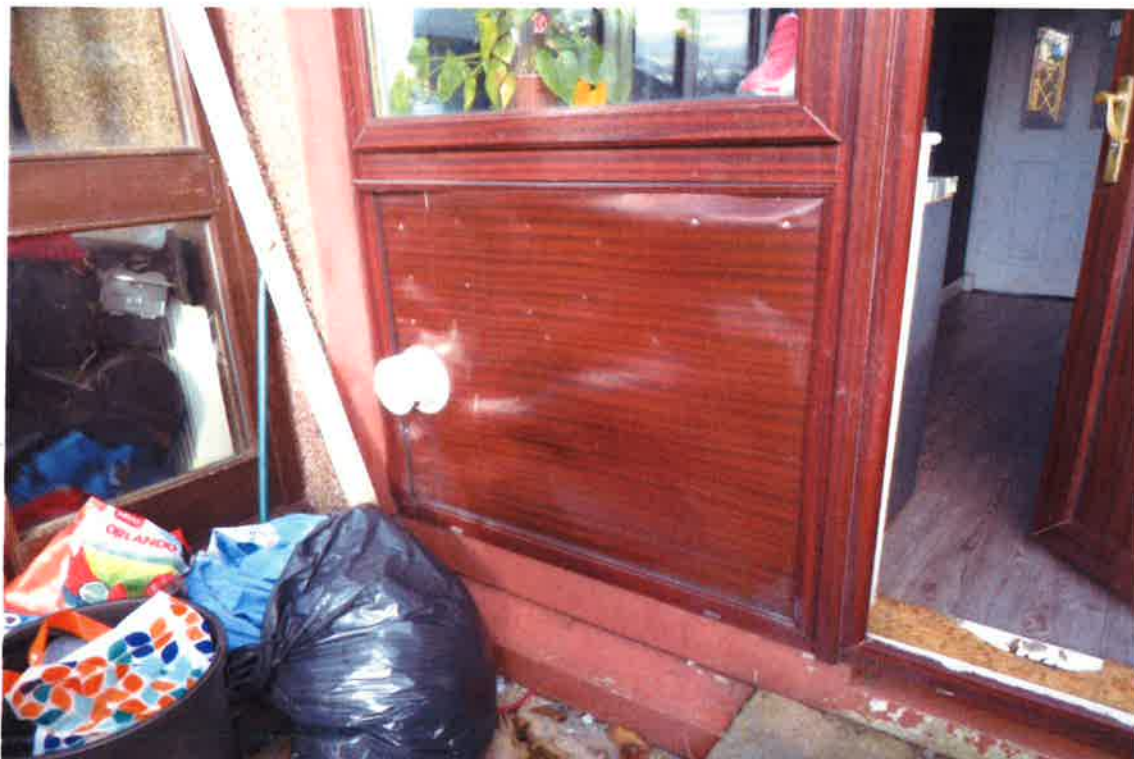
UPVC frame and inserted panel that requires repair / replacement
