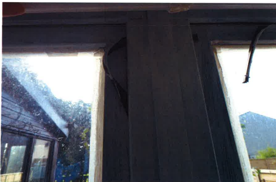
Sitting room window showing missing seals
