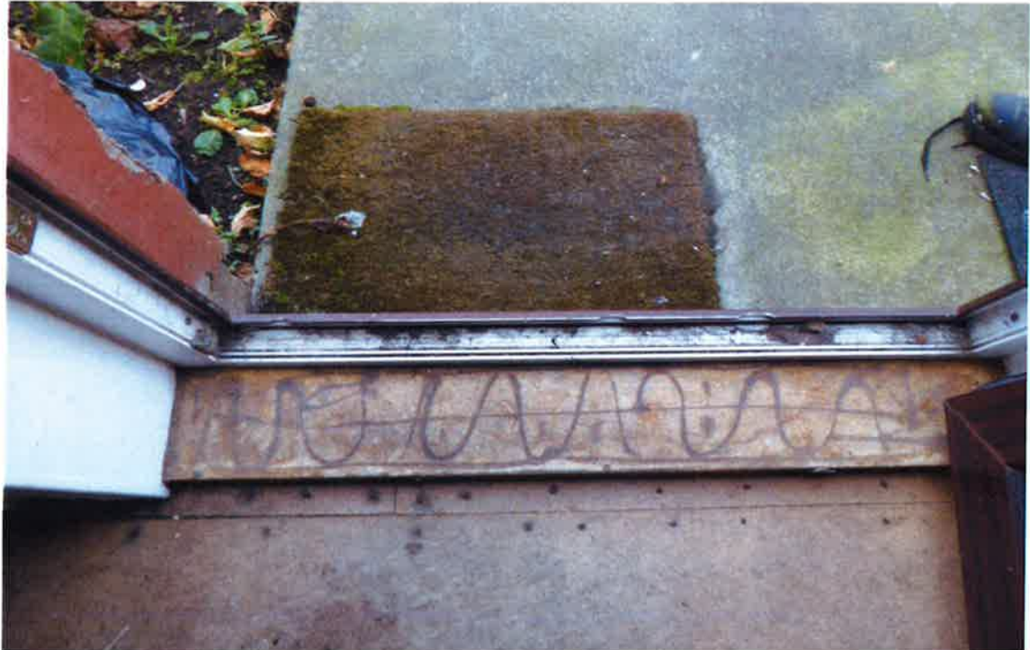
Front door showing damaged sill
