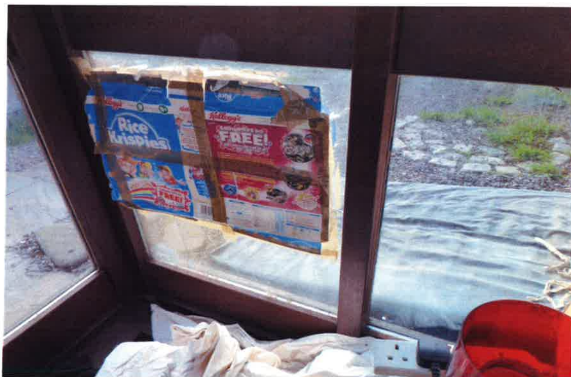
Cracked window pane
