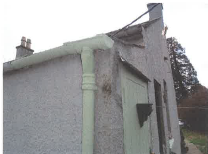
Repaired rain water goods and surrounding rendering 28 January 2020
