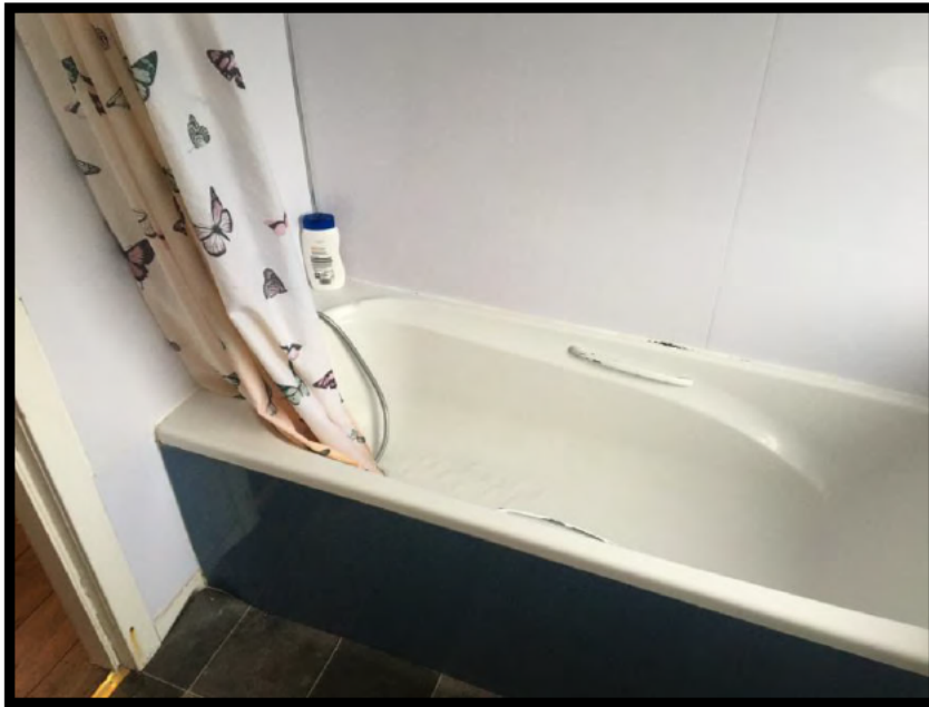
Photograph 18 - Bathroom - new waterproof linings around bath.
