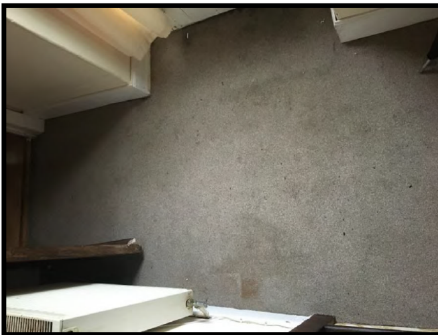
Photograph 6- Ground floor entrance - new carpet fitted by tenant.
