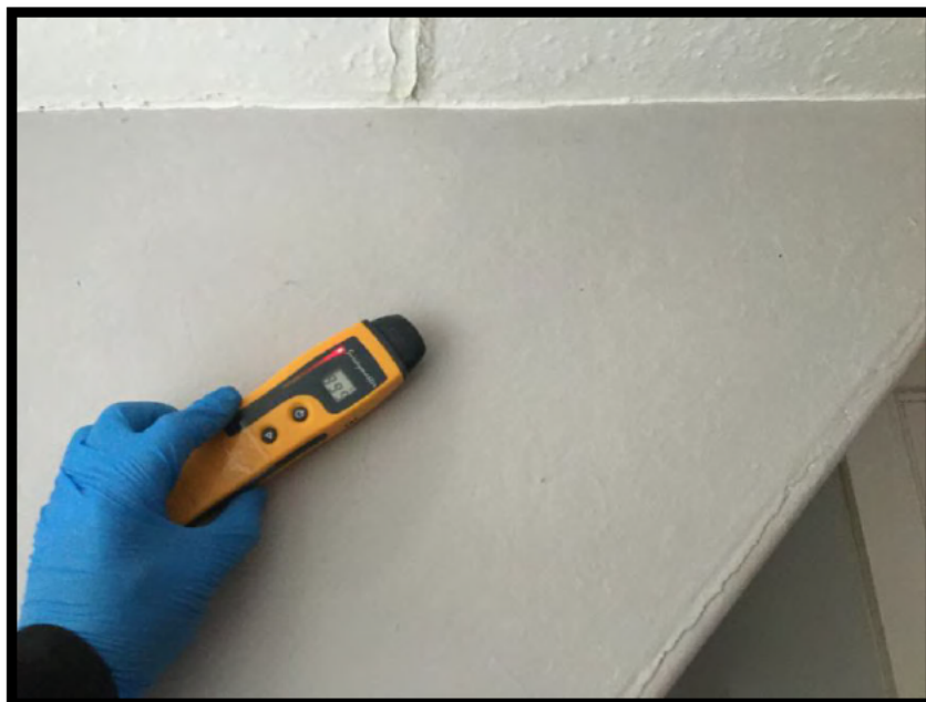
Photograph 12 - Moisture meter reading red (99%, three areas) to side of window dormer, left hand bedroom, unchanged
