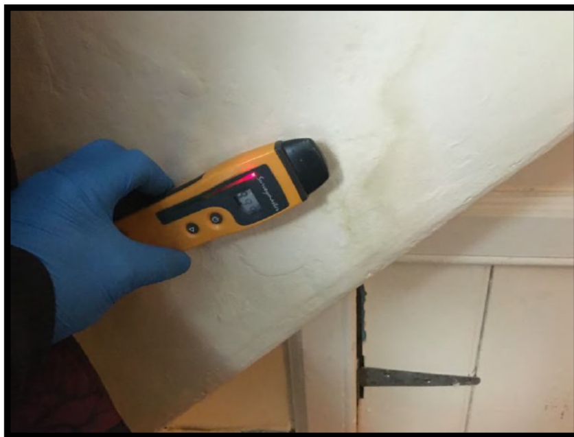
Photograph 10 - Moisture meter reading red (99%) to side of window dormer, right hand bedroom - unchanged.
