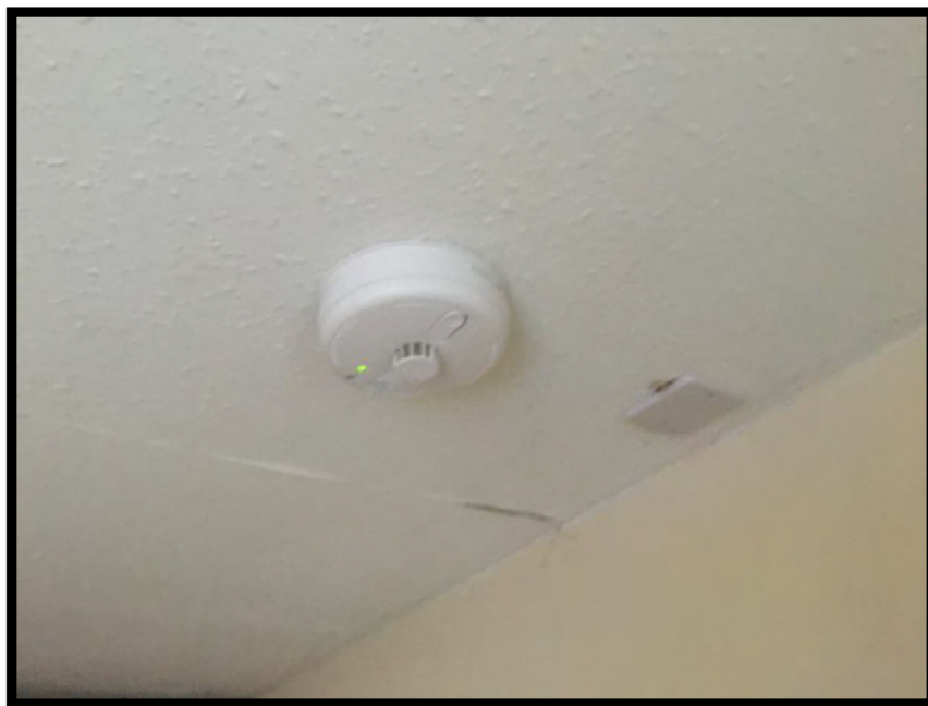
Photograph 2 Ground floor - Kitchen - Example hard wired alarm, alarm system tested at inspection.
