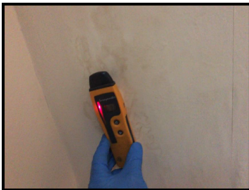
Photograph 11 - Moisture meter reading red (89%) to rear roof slope, right hand bedroom, previously green, 9%.
