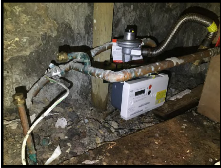
Photograph 12 - Gas meter cupboard - internal - unchanged.
