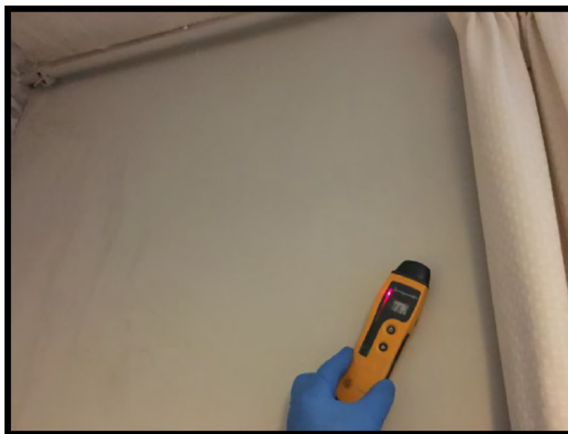
Photograph 8 Moisture meter reading red (96% localised spot) to front wall of sitting room - unchanged.
