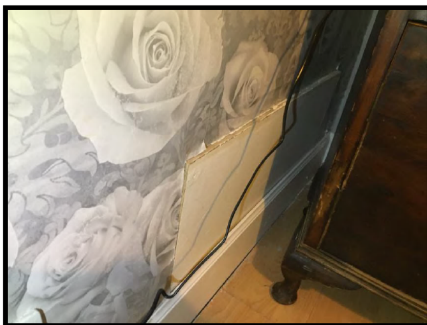
Photograph 11 - Gas meter cover, sitting room - unchanged.
