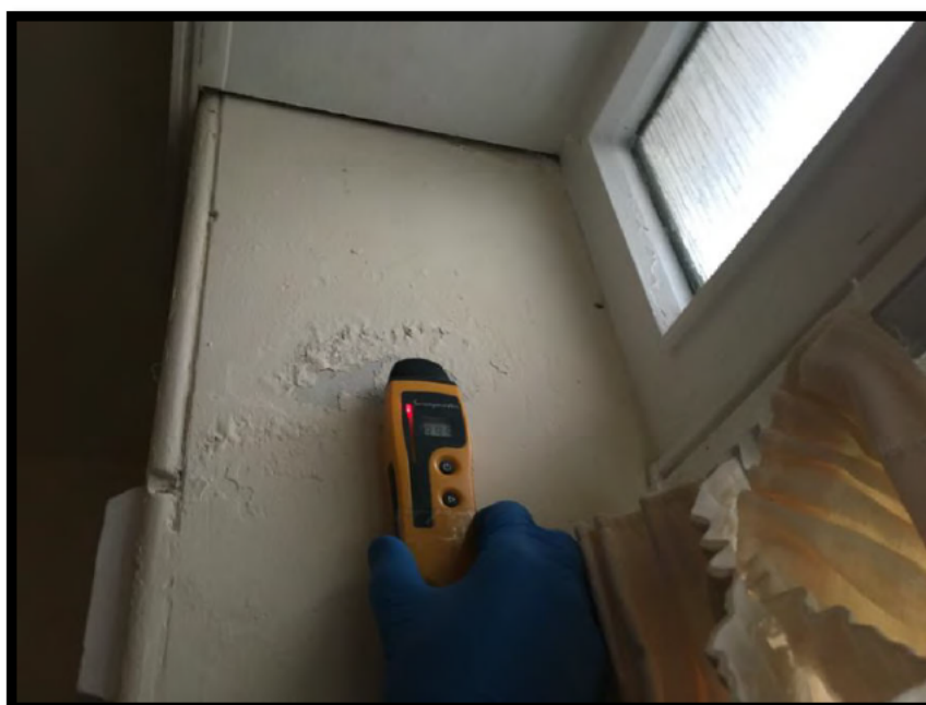
Photograph 9 - Moisture meter reading red (99%) to front wall at ground floor entrance. Both sides of door affected - unchanged.
