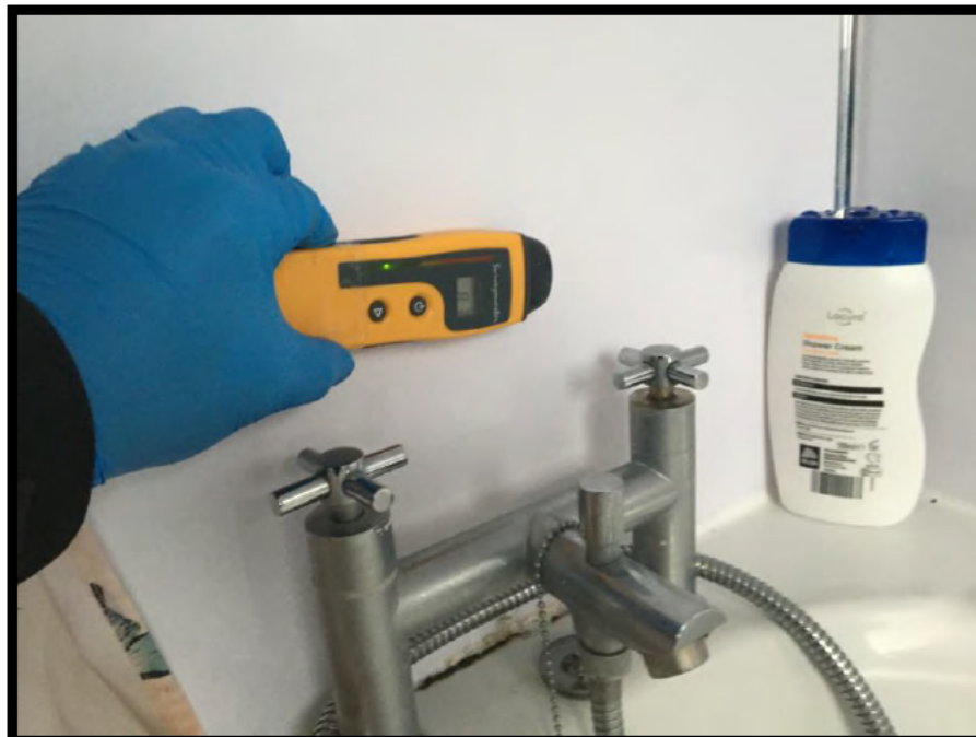
Photograph 17 - Moisture meter reading green (8%) to tiling at bath - was 99%.
