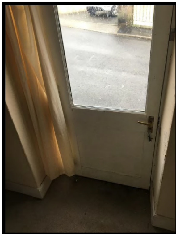
Photograph 3 Overview of front door - no significant change.
