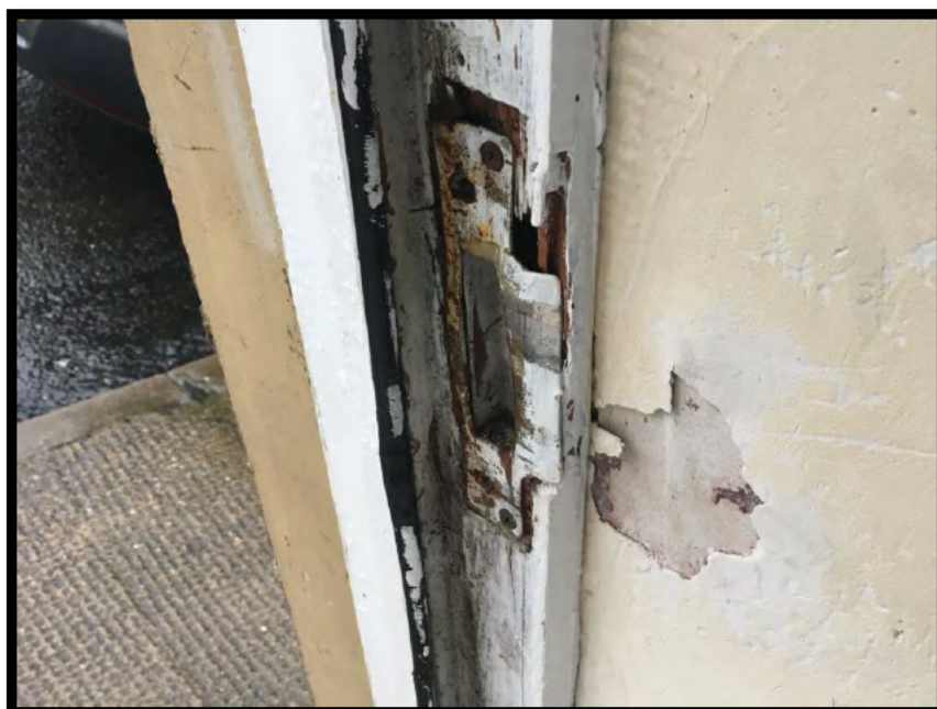
Photograph 5 Damaged lock keep - unchanged.
