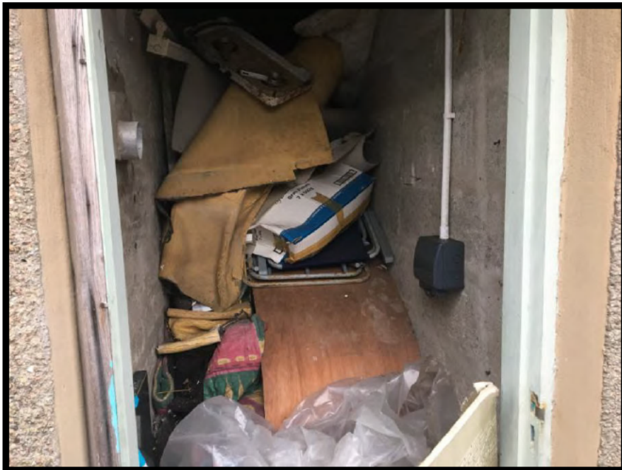
Photograph 13 External store attached to kitchen. Door missing, as before. Exposed electrical switch replaced with exterior style fitting.
