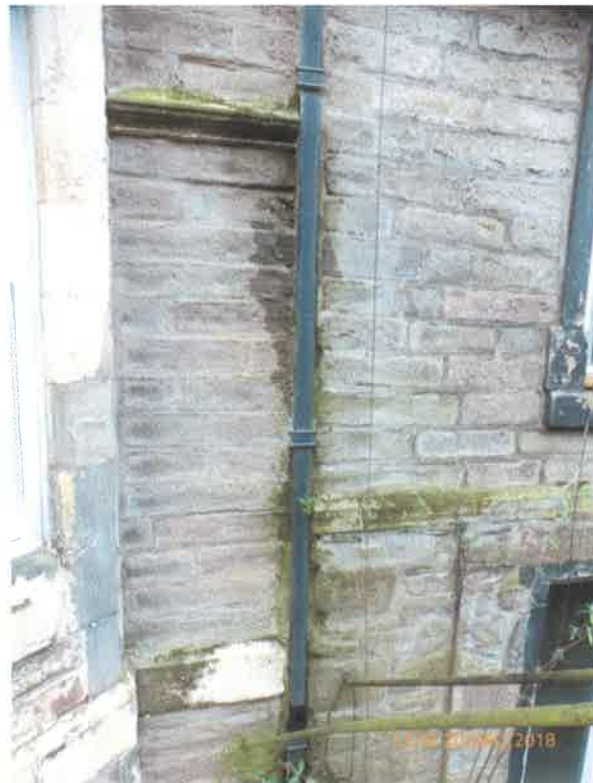
Leakage on front wall
