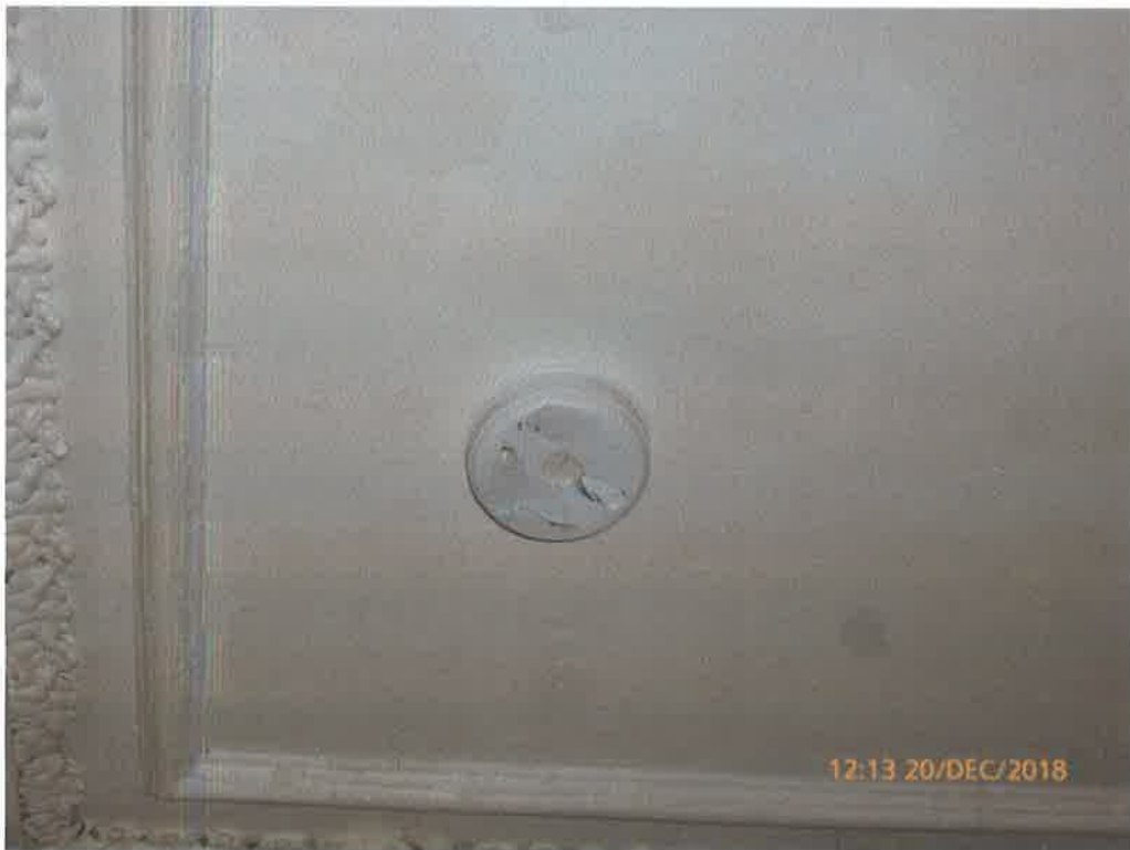
Broken heat detector
