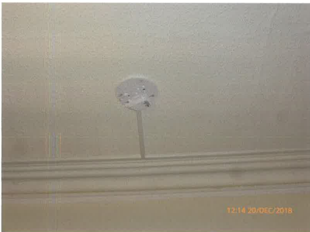
Missing smoke detector
