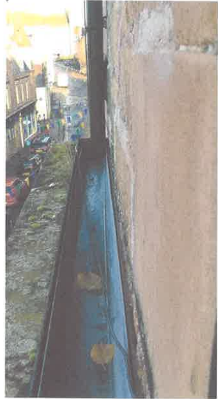
Photo 7 Gutter detail looking North
