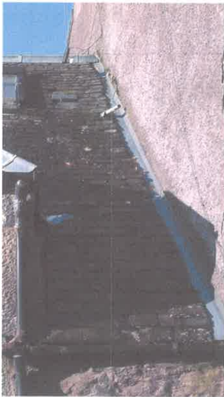
Photo 8 Roof detail on rear elevation
