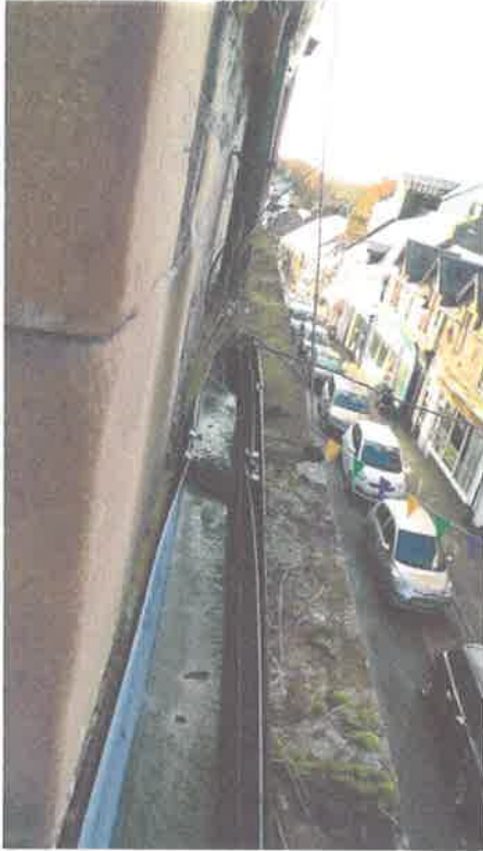
Photo 6 Gutter detail looking South
