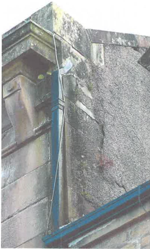
Photo 10 Adjoining gable detail to the North
