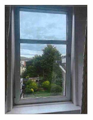
Windows have been fitted with trickle ventilation and new gaskets - no evidence of draughts or water ingress.
