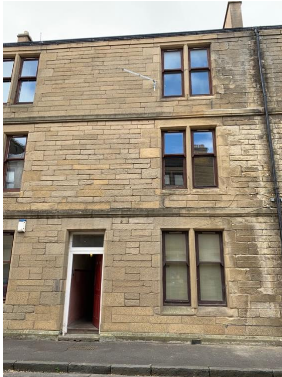
Photograph 1: Front elevation (ground floor)
