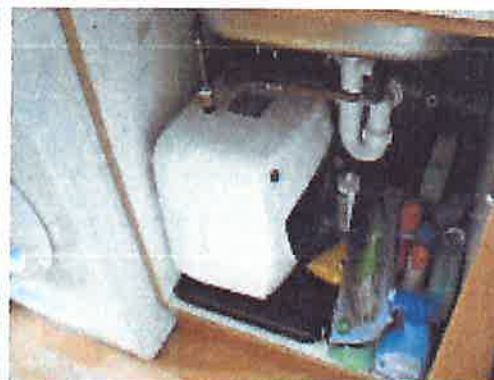
8. HOT WATER BOILER UNDER KITCHEN SINK
