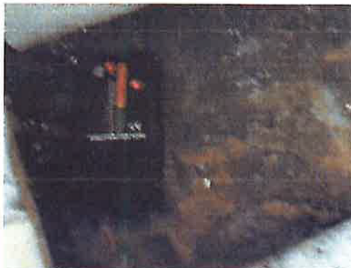
4. HIGH LEVEL OF DAMPNES IN FLOOR BESIDE WC
