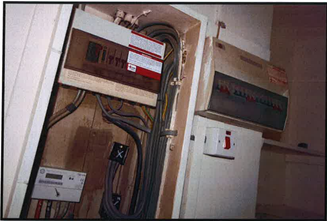
Figure 14 Electrical switchgear - right hand consumer unit no longer in use.
