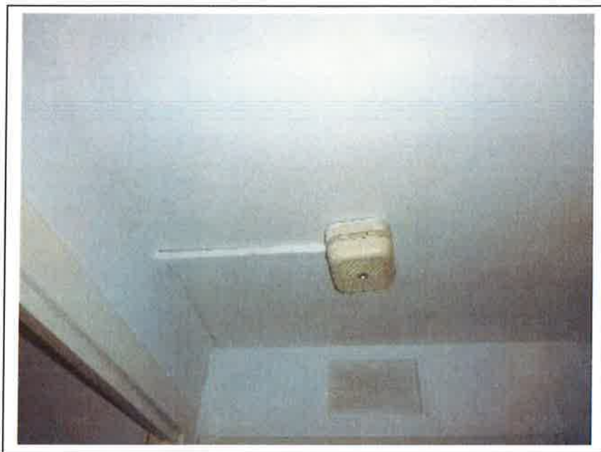
Smoke Detector in living room and another in the upstairs hallway.
