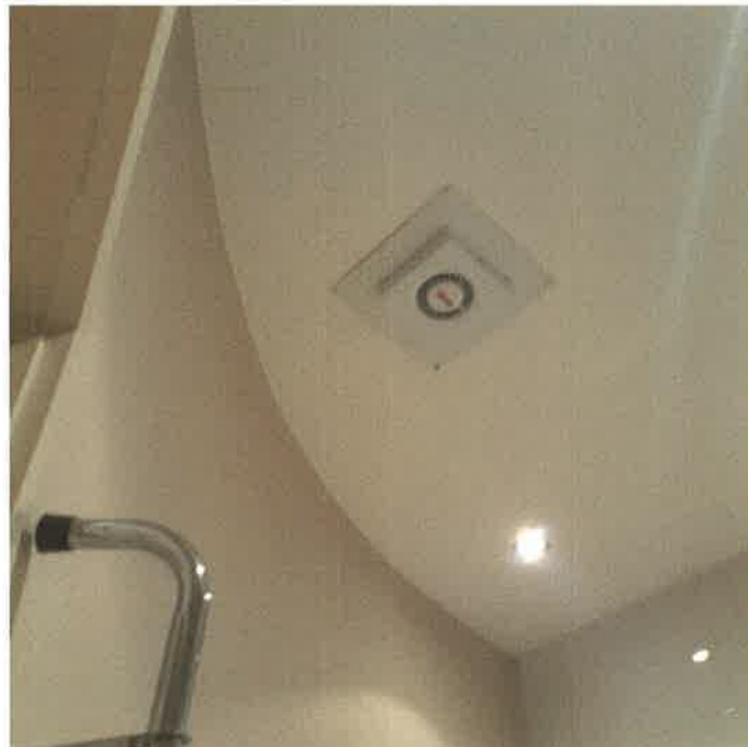
4 The new extract fan in the bathroom
