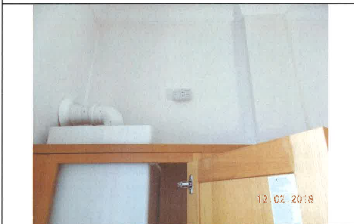
6. Carbon Monoxide Alarm
