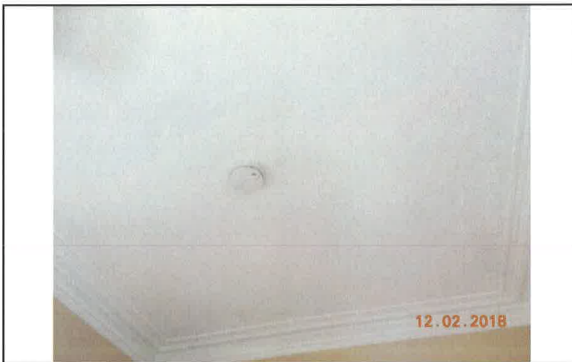
7. Smoke detector/alarm in hall
