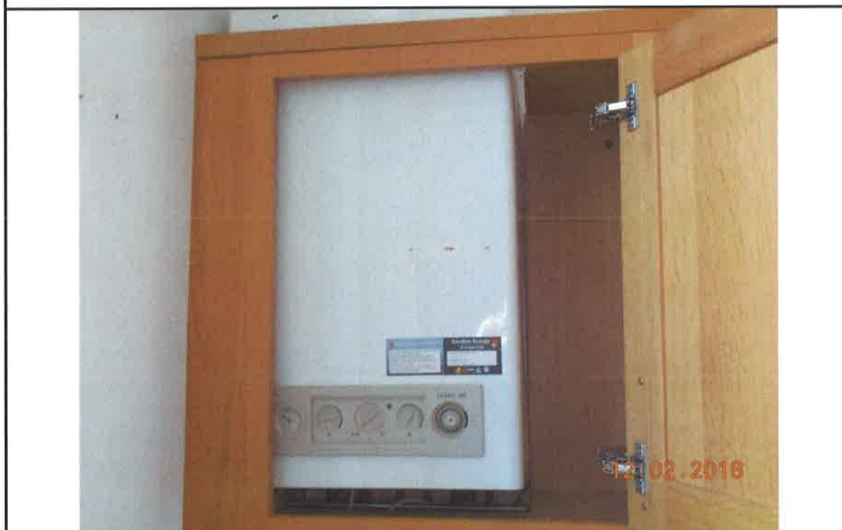
2. Gas fired central heating boiler
