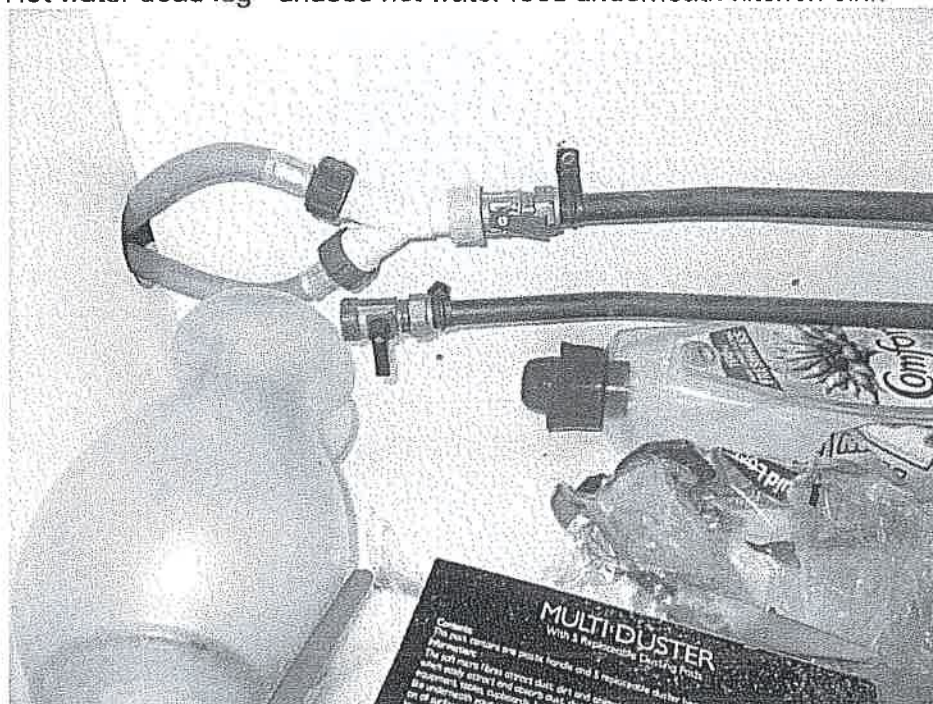
Hot water dead leg - unused hot water feed underneath kitchen sink
