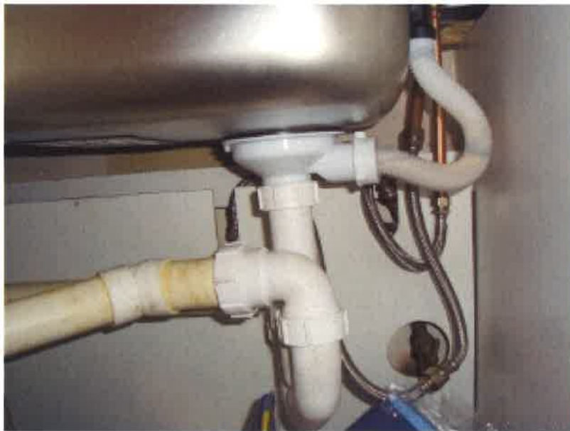
"DEAD LEG" PIPE REMOVED-KITCHEN SINK
