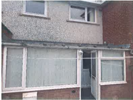
Rear Entrance porch with glass roof. Flashing detail repaired.
