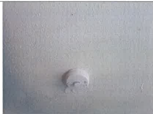
Combined smoke and heat detector
