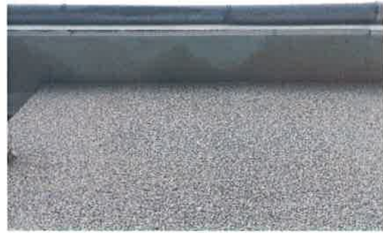
Guttering repaired at front and rear, damp staining noted to boarding.
