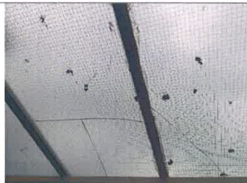
Cracked glass roof panels in porch. No water ingress. Surrounding areas were dry at time of inspection
