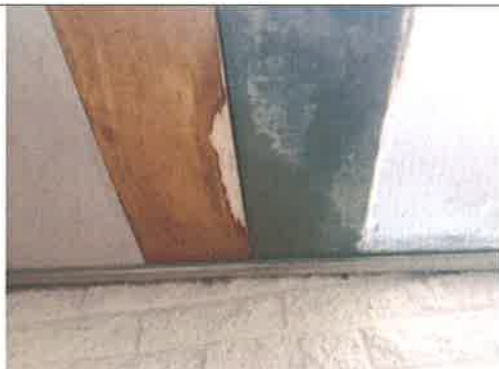
Repaired porch roof. Dry at time of inspection. Externally repaired with a flashing detail.
