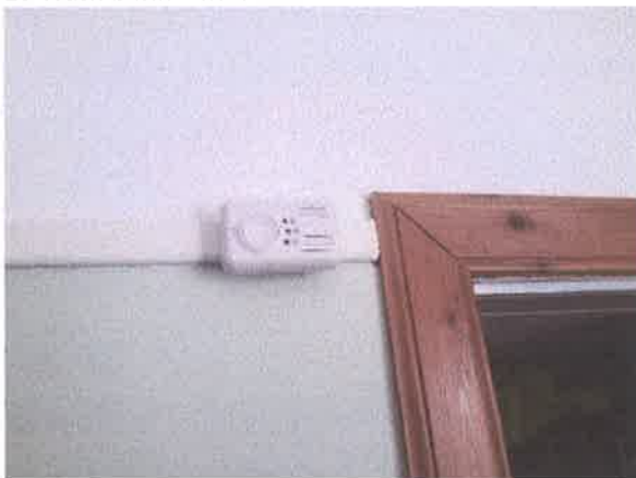
15 Carbon Monoxide alarm
