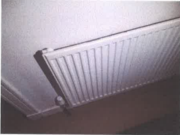
9 Central Heating installation.
