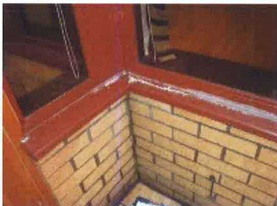
REPLACED TIMBER SILLS, EXTERNAL AND INTERNAL – CONSERVATORY
