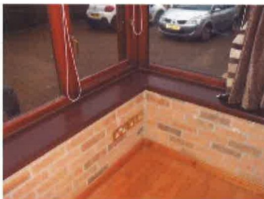
REPLACED TIMBER SILLS, EXTERNAL AND INTERNAL – CONSERVATORY
