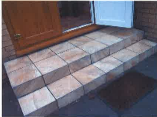
ENTRANCE PORCH- INT SILL REPAIRED. NEW TILES AT ENTRANCE STAIR
