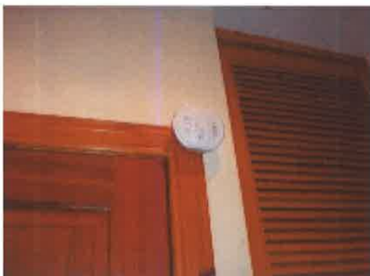
CO MONITOR AT BOILER
