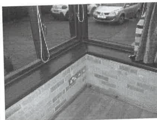
REPLACED TIMBER SILLS, EXTERNAL AND INTERNAL – CONSERVATORY
