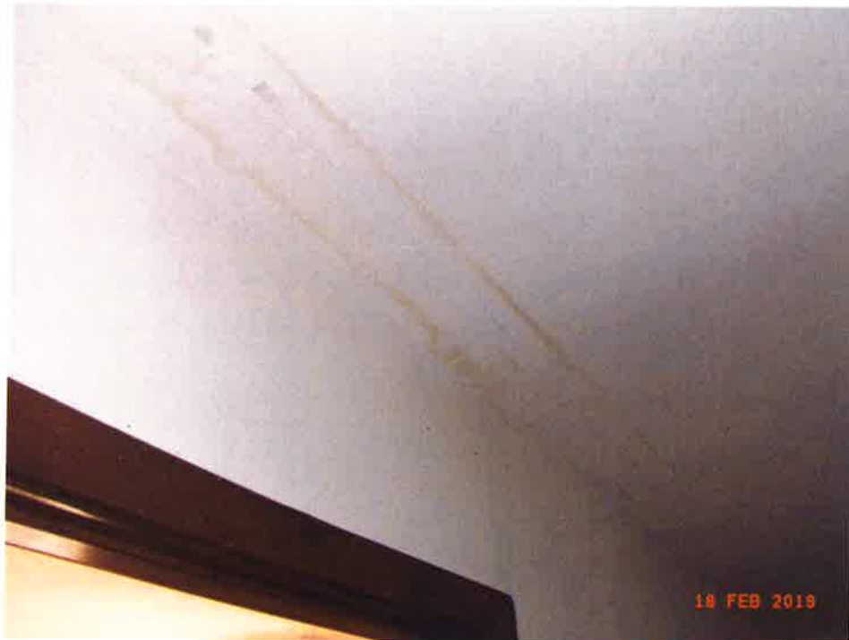
Damp staining on Utility Room ceiling. (1)
