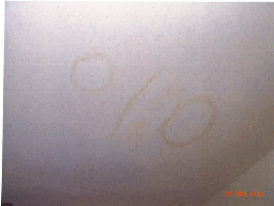
Damp staining on Utility Room ceiling. (2)
