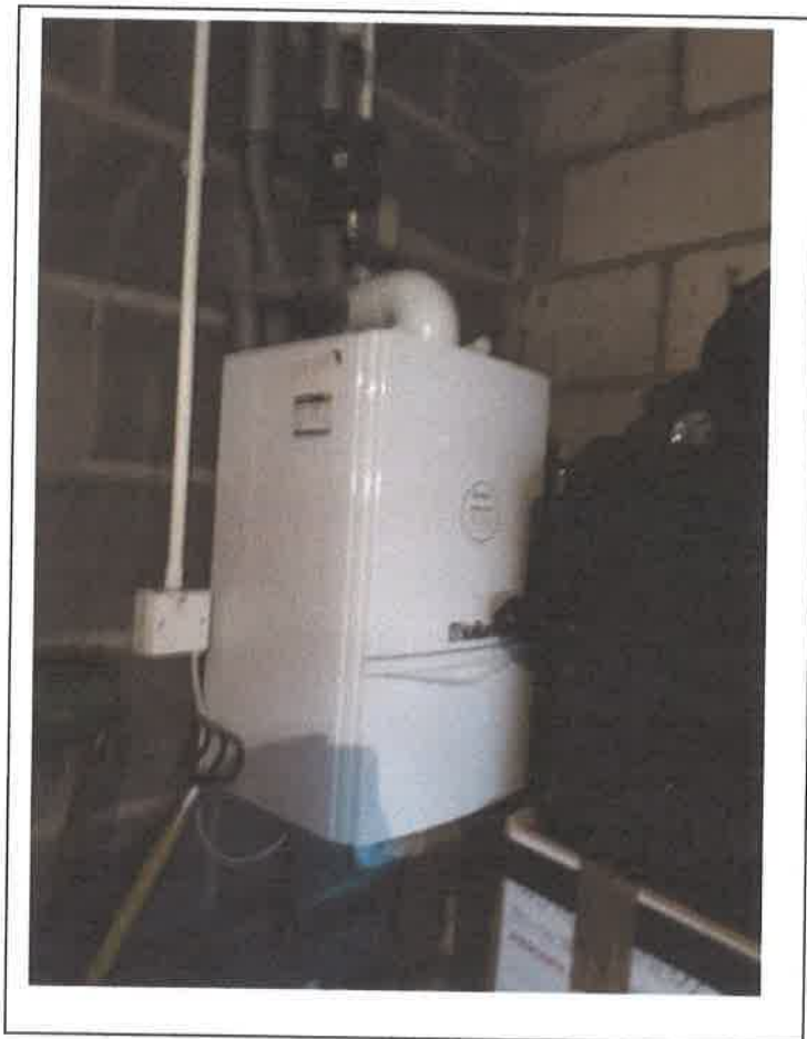
Gas Central Heating boiler located within the integral garage – No Carbon Monoxide monitor
