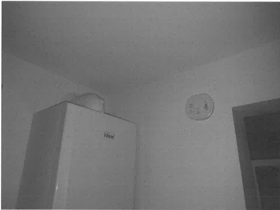
5 Carbon Monoxide detector.
