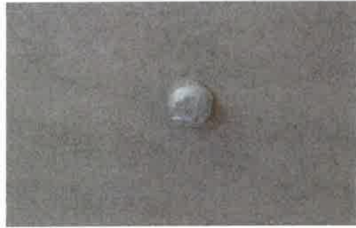
Photo 5 – Smoke detector in hall
