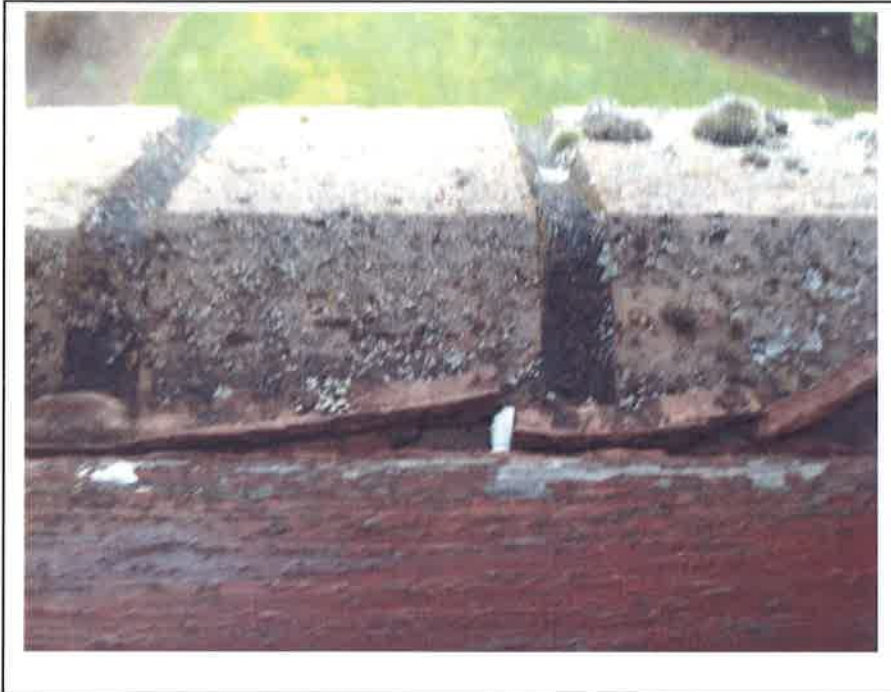
Windows weathered and mastic spalling. Maintenance required.
