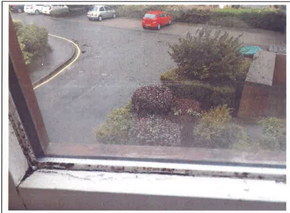
Windows weathered and mastic spalling. Maintenance required.
