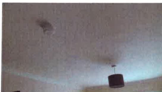
Photo 8 – Operative living room alarm
