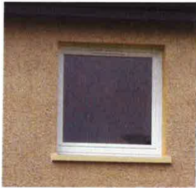
Photo 2 – New windows throughout
