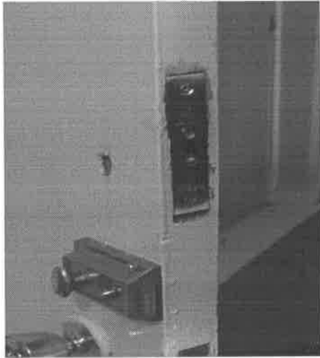
Photo 3 Replacement door lock
