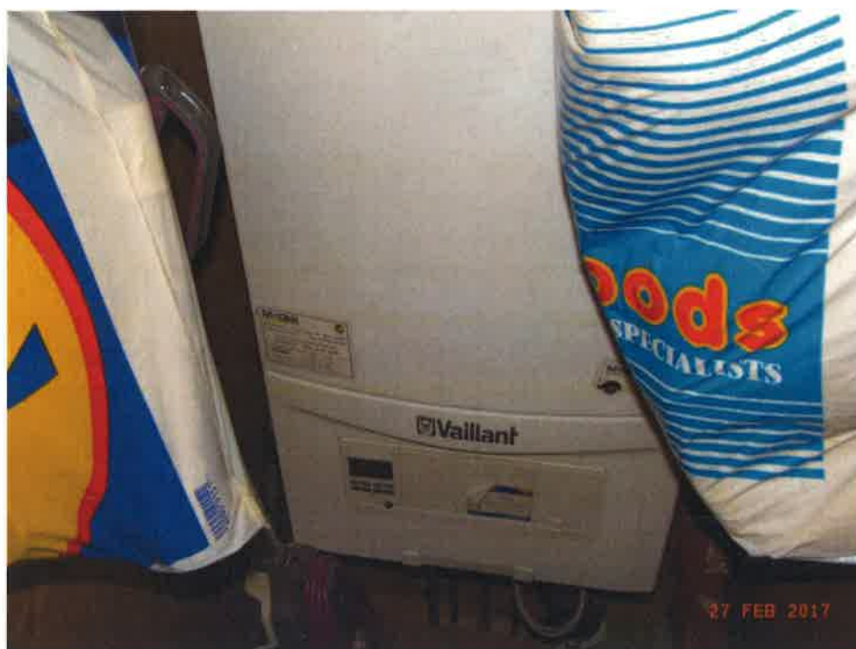
Central heating boiler
