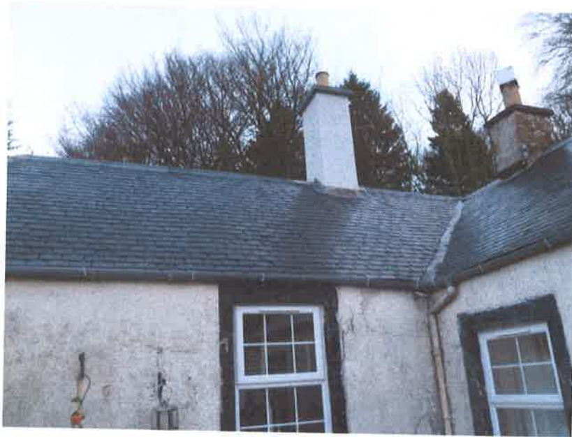
9. Roof showing slipped slates. Gutters realigned.
