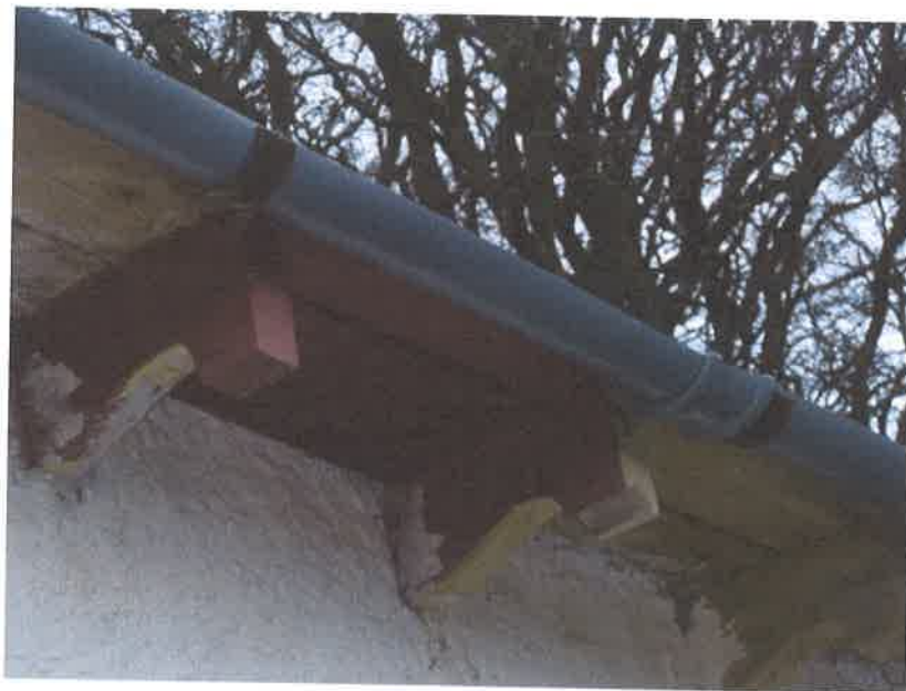
10. Repair to hole in eaves soffit
