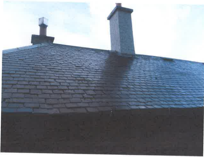
11. Roof showing slipped slate
