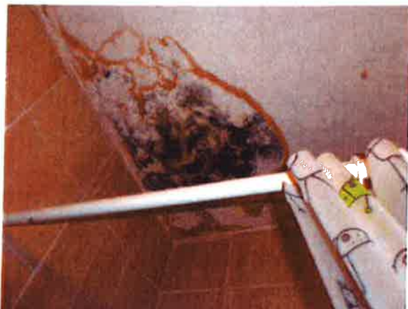
Water damage bathroom ceiling - November 2017
