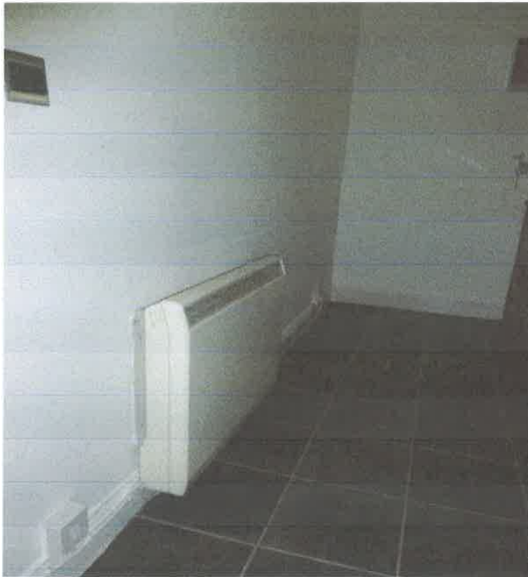
Kitchen – convector heater to wall
