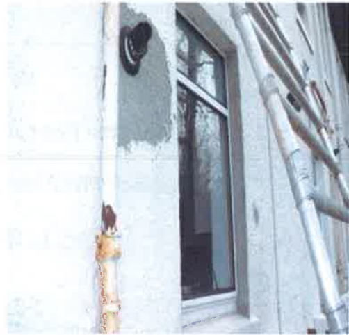
(Ph4) R/E – Roughcast repairs
