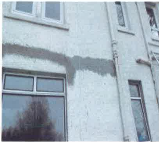
(Ph3) R/E – Roughcast repairs
