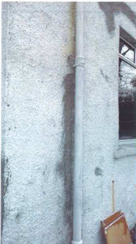
(Ph5) R/E – Roughcast repair
