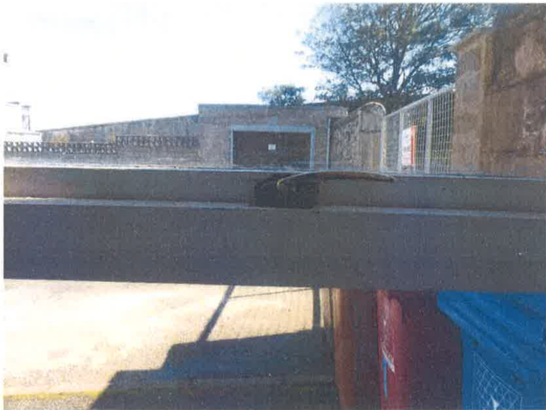
Front ground floor sitting room window – top section - catch
