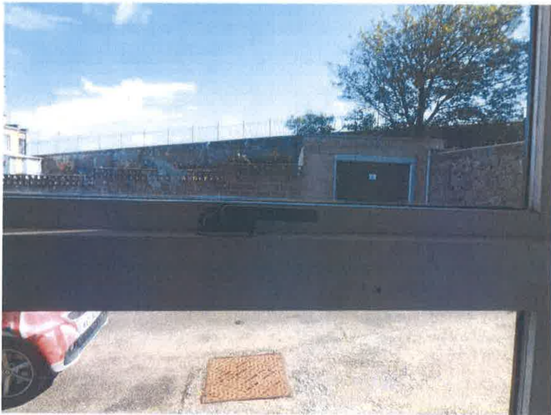
Front ground floor kitchen window – top section – catch
