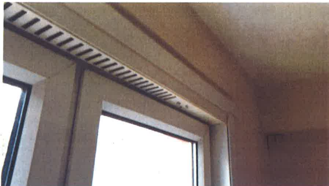
3 The repaired window vent
