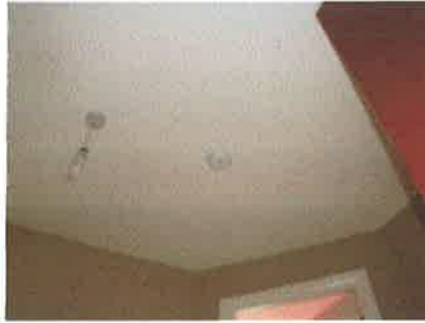
Smoke detector in Upper Landing.
