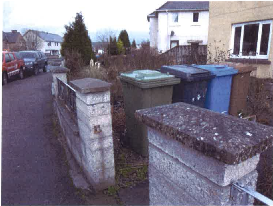
Photograph 2: Re-bed front gate coping stones- COMPLETED
