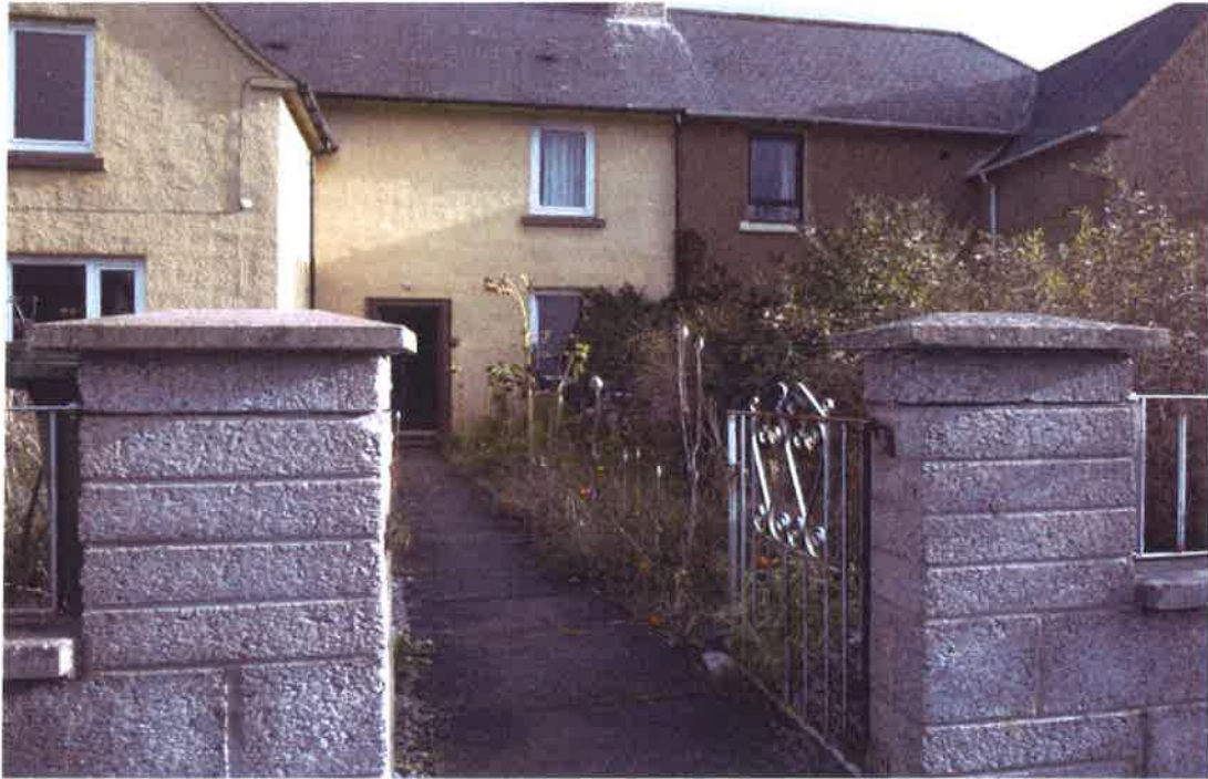
Re--bedded Coping stones at front of property
