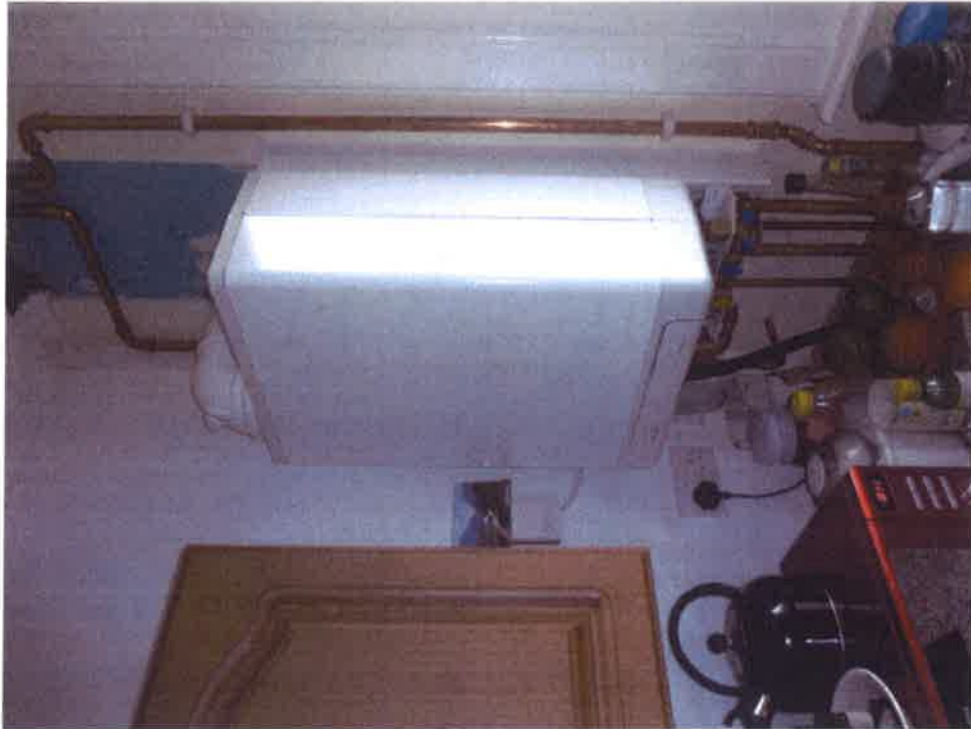
Photograph 4: Repair Central heating. New boiler installed. COMPLETED
