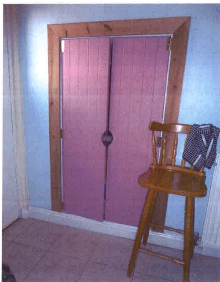
Kitchen alcove now reinstated and skirting boards fitted
