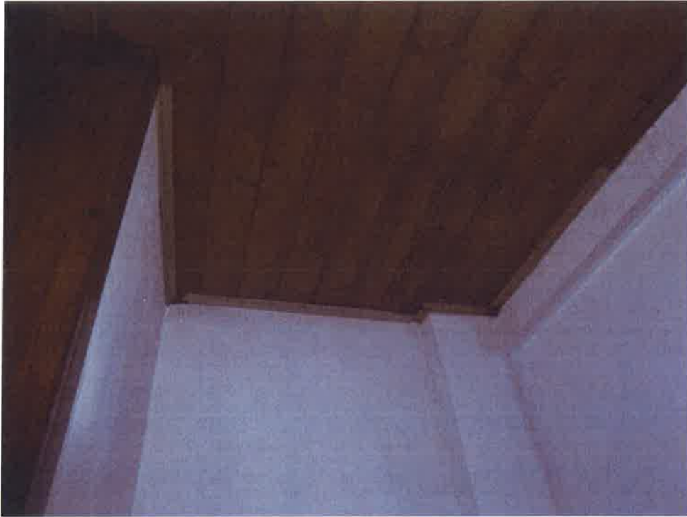
Photograph 10:: Quadrant bead to hallway ceiling. COMPLETED
