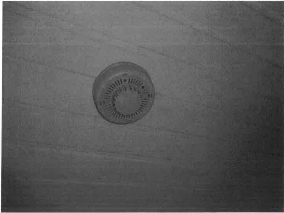
Kitchen ceiling – heat detector verified and working by Fire Service
