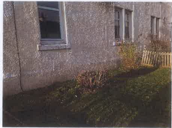
16 Patch repairs to Front Elevation.
