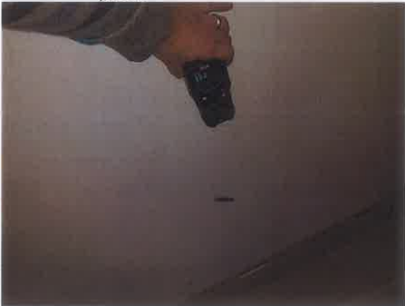
5 Acceptable moisture content in Bedroom.
