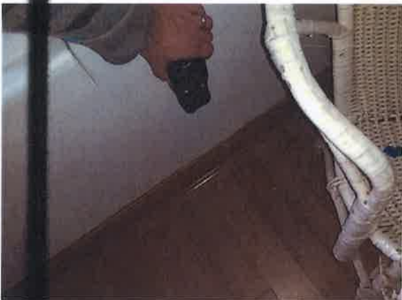
7 Acceptable moisture content at low level walls.
