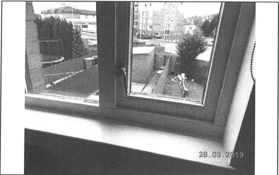
1. Handle to window now in place
