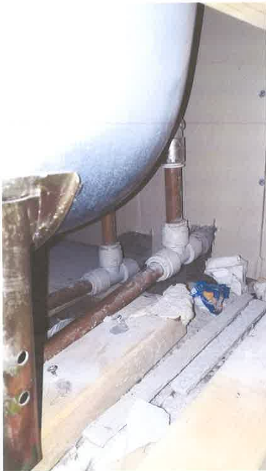
3 View of the secured pipe fittings below the bath
