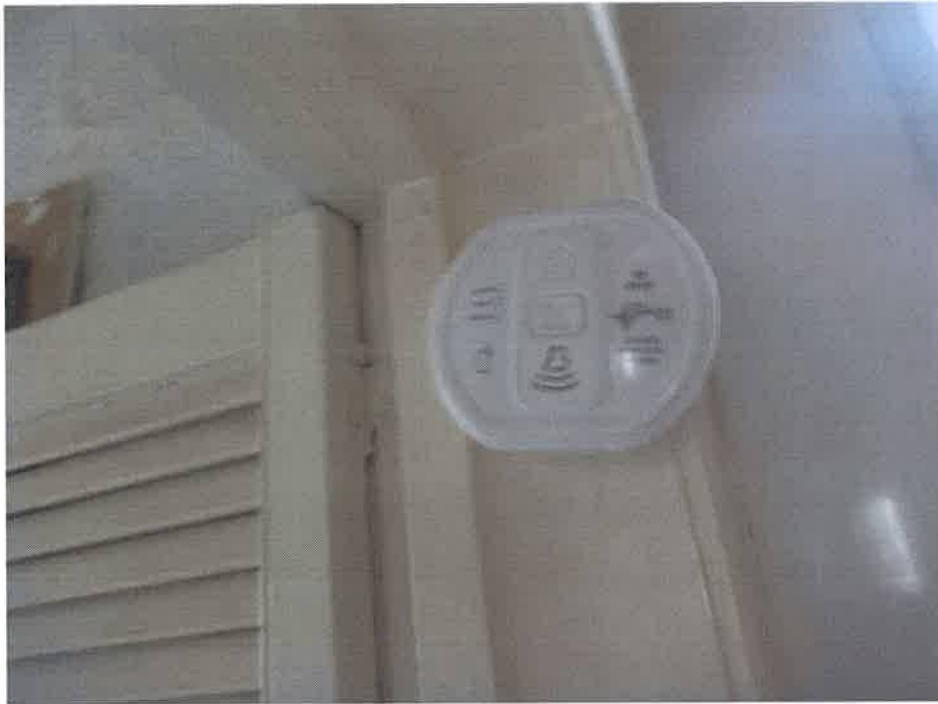
Carbon Monoxide monitor in position adjacent to boiler
