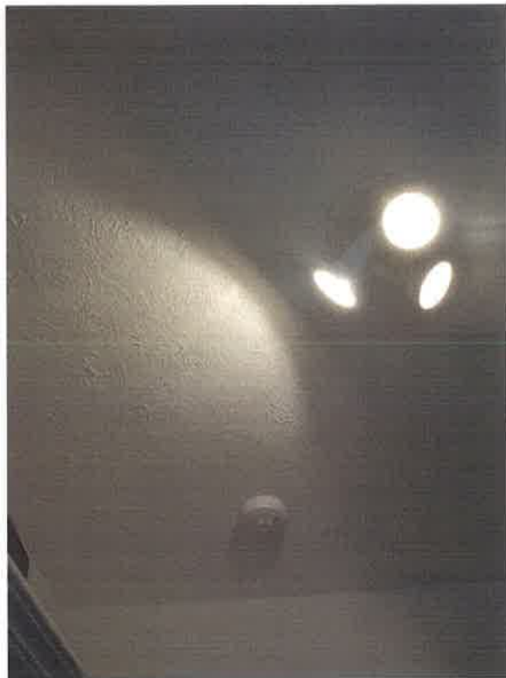
Smoke and heat detector located within the kitchen
