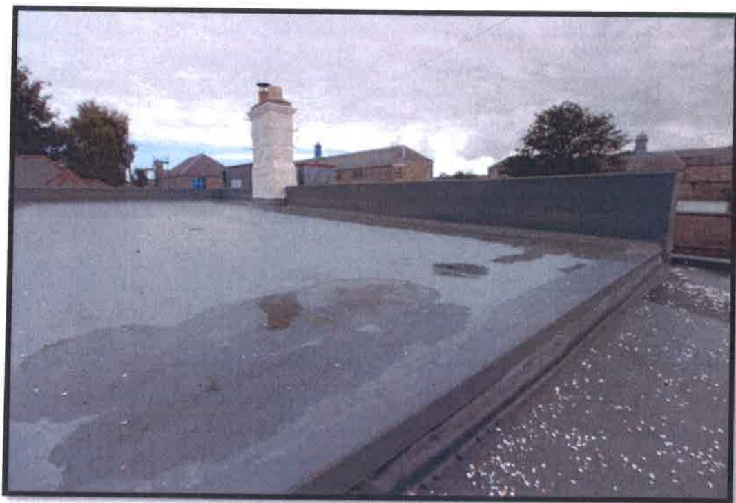
Figure 20 Rear section of flat roof at kitchen/utility room junction with some ponding over former kitchen, tears at junction with rear roof repaired.
