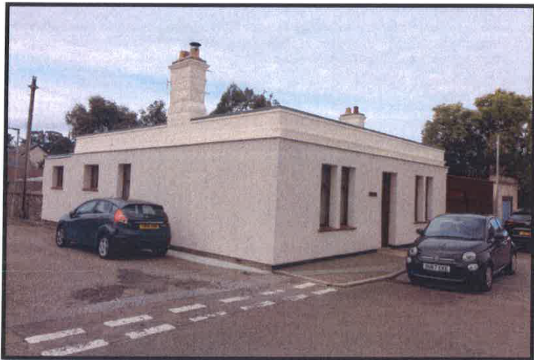
Figure 1 Front and side elevations, new insulated cladding present.
