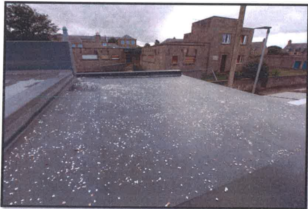
Figure 19 Rear section of flat roof over former utility room/new kitchen - now re-covered.
