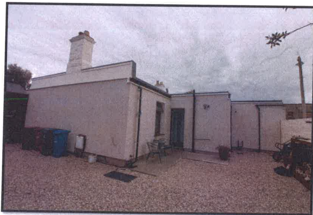
Figure 17 Rear entrance - new cladding and rainwater goods.
