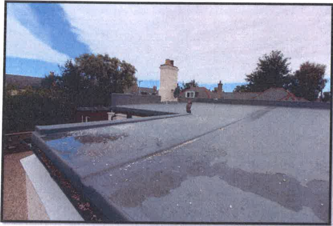
Figure 18 Rear section of flat roof with some ponding over bathroom, as before.
