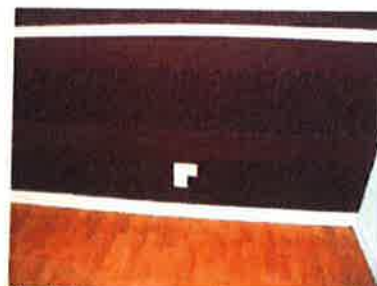
04 - Living room - power socket
