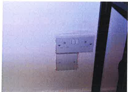
Living room power socket 29-10-18
