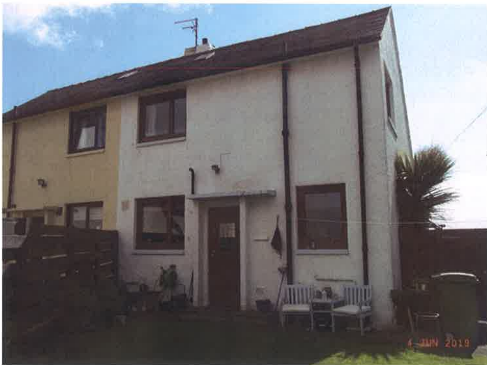
Rear elevation showing replacement windows
