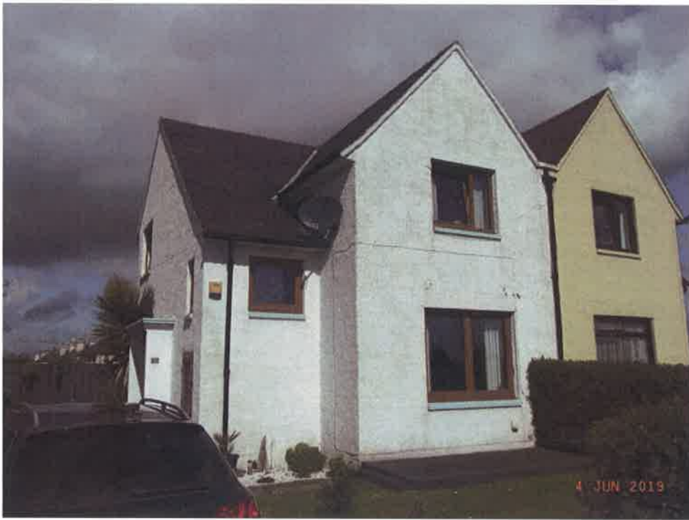
Front elevation showing replacement windows
