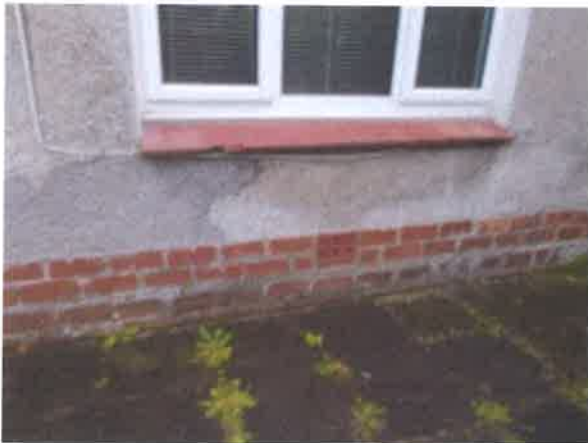
Rear Elevation showing base of external wall
