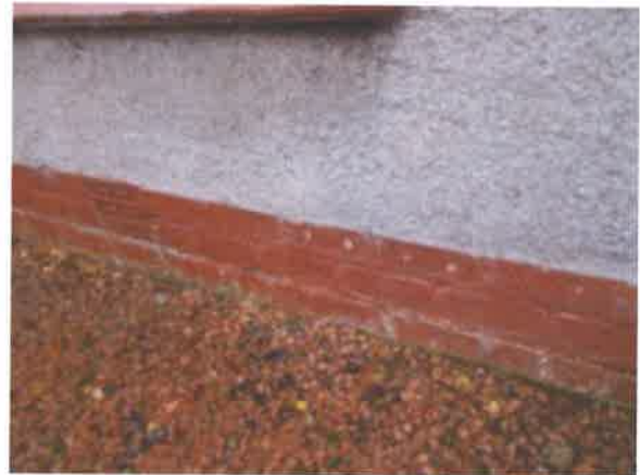
Front Elevation showing base of external wall
