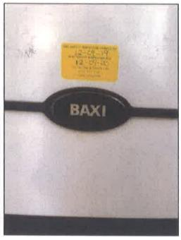
Carbon dioxide monitor fitted to cupboard housing the combi boiler. Combi boiler has had an up to date gas safety inspection carried out on the 12/09/19.
