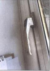
No evidence of condensation noted during inspection, slightly high reading of dampness on one section of flooring, this could be due to owner steam cleaning bathroom tiles. No extract fan noted but window opened and closed with ease and trickle ventilation is present.
