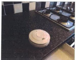
Heat detector unit in kitchen requires to be fitted to ceiling
