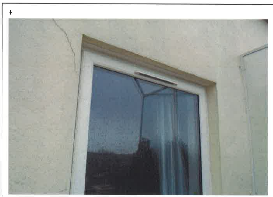
Replacement double glazed windows with trickle vents.
