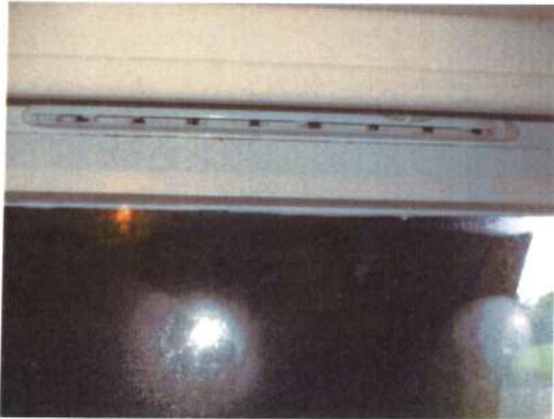
Bedroom Window Vent
